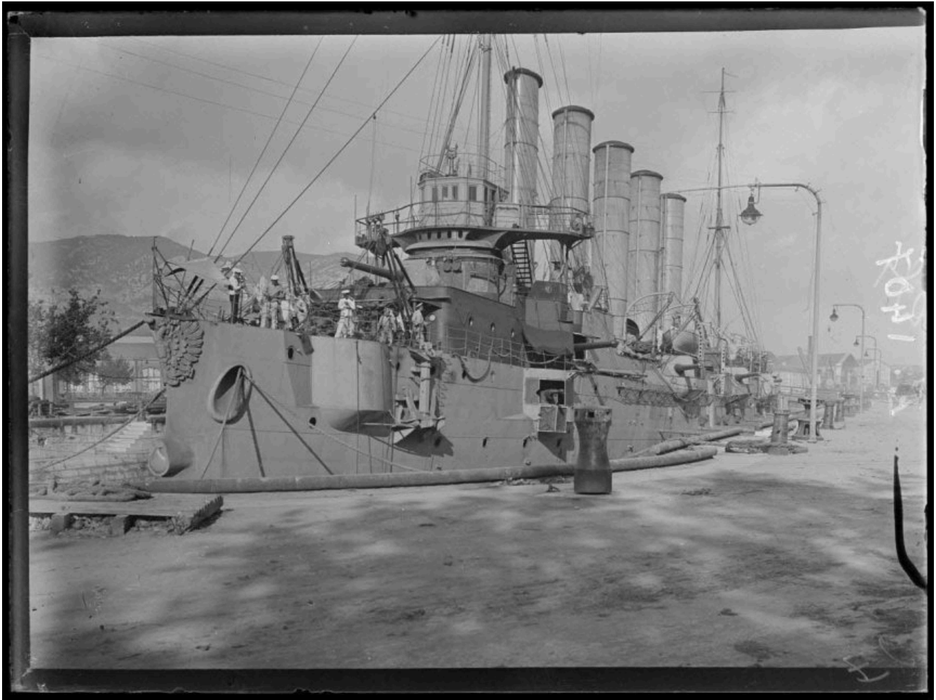
Russian protected cruiser Askold under repair in Toulon, Sept 1916
